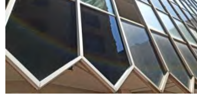
Zurich Building, Barcelona
